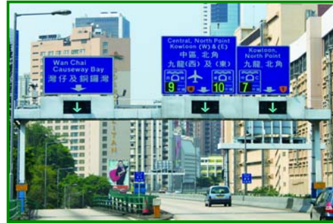
2 Canal Road Flyover northbound (near exit of Aberdeen Tunnel)
