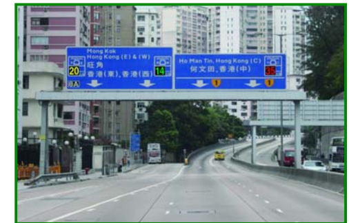
7 Waterloo Road southbound (near Kowloon Hospital)
