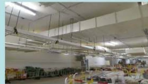
安裝風槽及電纜管道 Ductwork / Cable containment Installation
