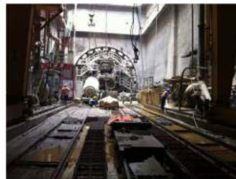
深圳段 - 皇崗豎井底工況 Shenzhen section - Progress at Huanggang Shaft
