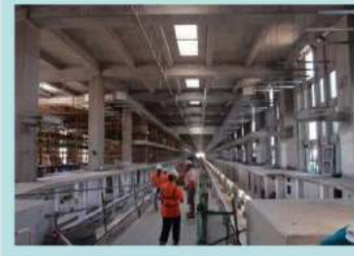
列車維修大樓內部 Internal view of Running Maintenance Shed
