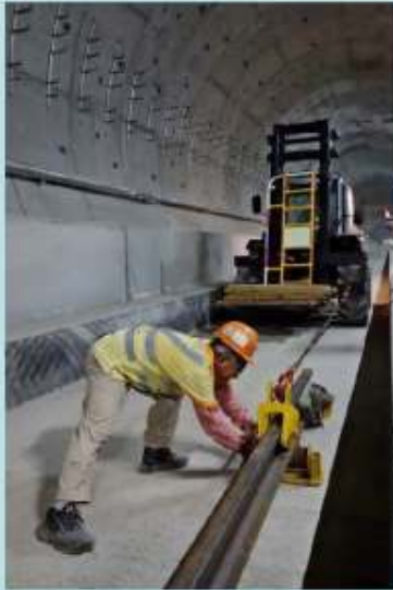
鋪設路軌 Track laying
