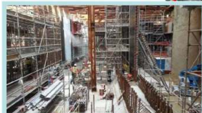
旺角西通風樓建造工程 Mongkok West Ventilation Building Construction
