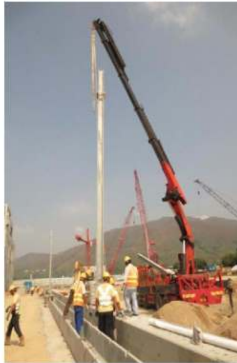
豎立高架接觸網支柱 Overhead Line Mast Erection
