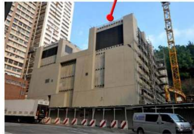
葵涌通風樓 Kwai Chung Ventilation Building
