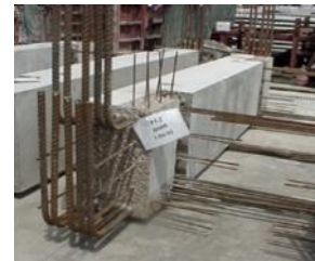
Precast Tie Beams
