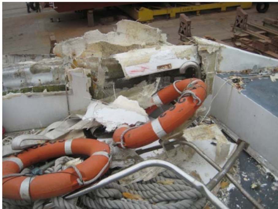
Figure 4: Photo showing the extent of damage to the part of Sea Smooth involved in the collision
