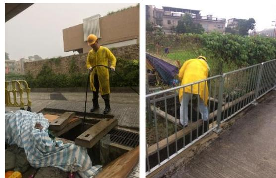
Workmen thoroughly cleared the storm water drains near the downstream farmland area to keep the drainage system clear from blockage.
