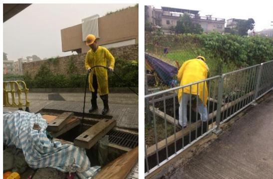
Workmen thoroughly cleared the storm water drains near the downstream farmland area to keep the drainage system clear from blockage.
