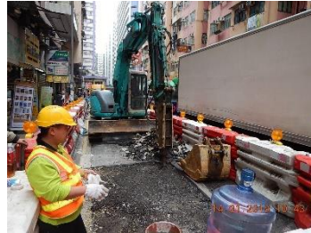
Cheng and his team had to excavate the road surface to replace the defective sewer located six metres underground.
