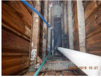
Cheng and his team had to excavate the road surface to replace the defective sewer located six metres underground.
