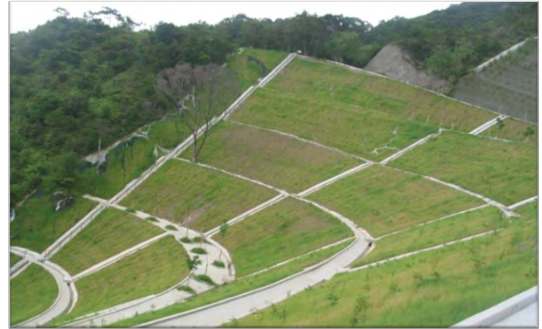
Enhancement of slope drainage capability
