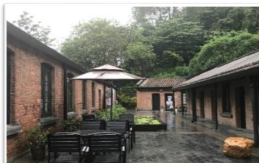
前荔枝角醫院 (饒宗頤文化館) Former Lai Chi Kok Hospital (Jao Tsung-I Academy)
