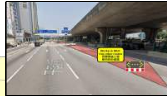
干諾道西 (西行) Connaught Road West (Westbound)
